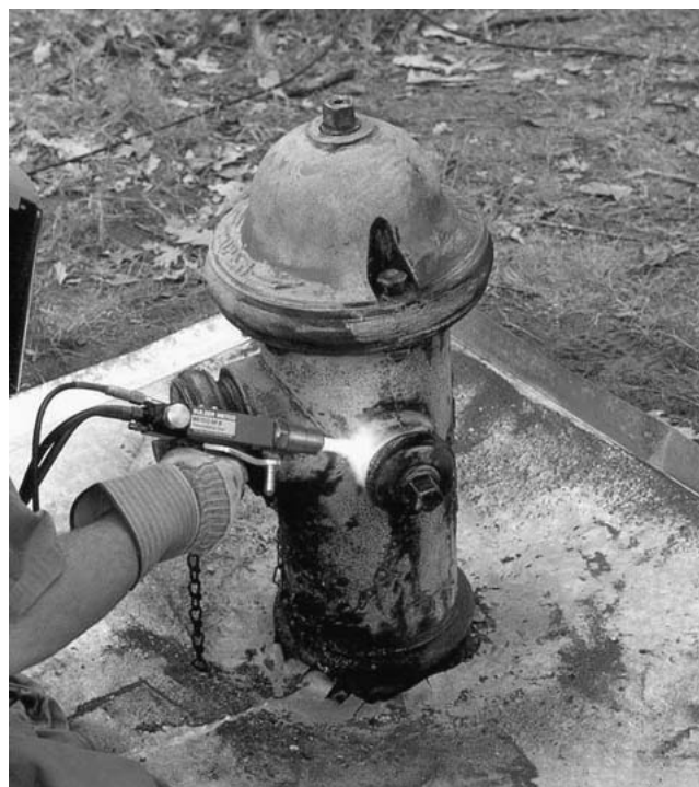
Fig. 2 TSV process on Fire hydrant at Fort Drum to remove lead-containing paint
